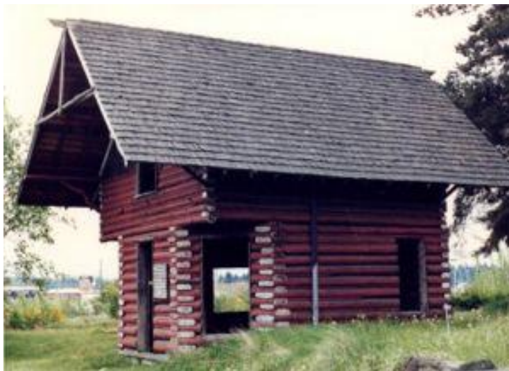
The David T. Denny Cabin before restoration
