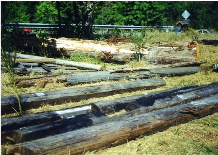
Fig. 25 – Original sidewall logs and new cedar log being sorted prior to Barker Cabin restoration, September, 1999. (Courtesy Lynda Jenkins, HSFW.)
