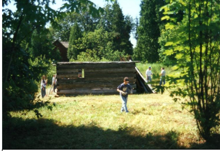
Fig. 22 – The small single window is shown here on the north side of the cabin. This window is now on the cabin’s south side, October 2, 1997. (Courtesy HSFV.)
