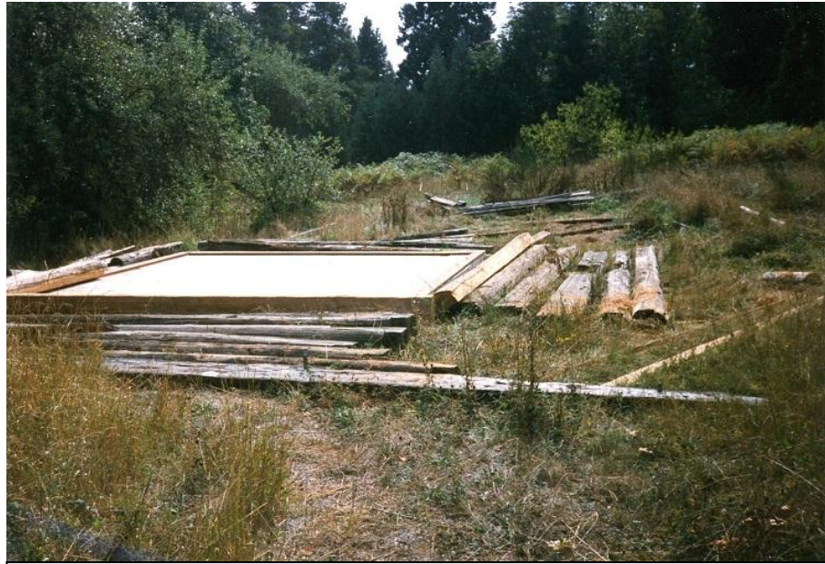
Fig. 26 –The original sidewall logs for the Barker Cabin arranged and in place for the second restoration, September 23, 1999. (Courtesy HSFW.)
