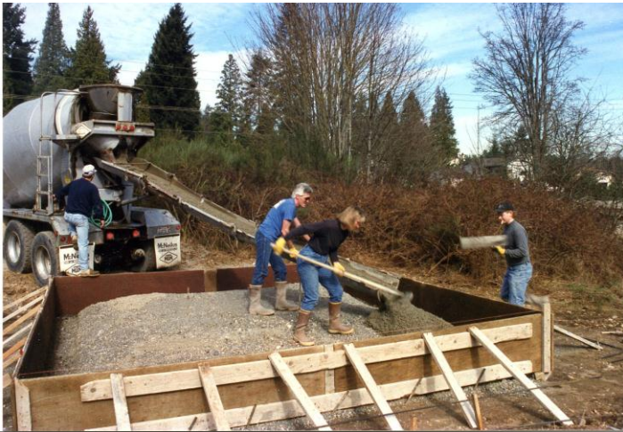
Fig. 17 – J & K Foundations pouring Barker Cabin slab, May 24, 1994. (Courtesy HSFW.)
