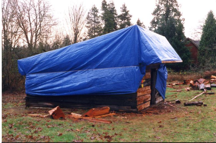
Fig. 29– Partially restored Barker Cabin covered with a blue tarp for protection from the weather, November, 1999. (Courtesy HSFW.)
