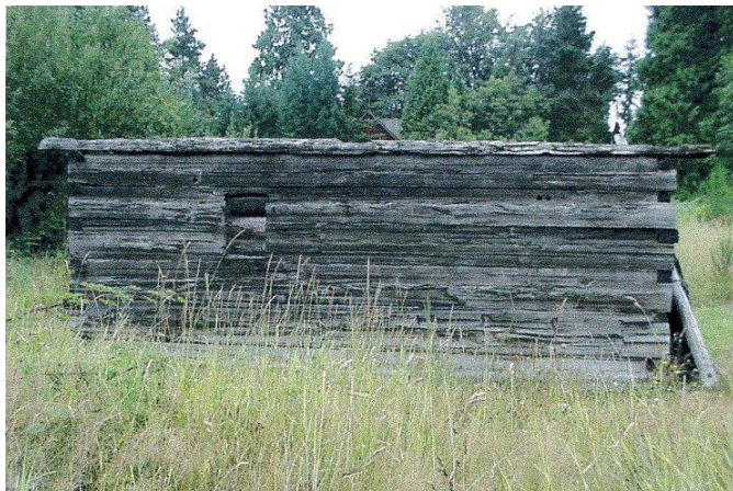
Fig. 21 – Temporary reassembly of sidewalls, with the small single window on the north side of the cabin, Circa mid 1990s. (Courtesy HSFW.)
