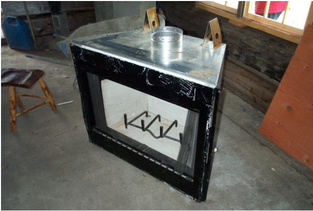
Fig. 42 – The metal firebox for the fireplace in the Barker Cabin, 2008. (Courtesy HSFW.)
