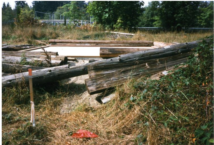
Fig. 19 – Original logs placed on ground by the side where they would be erected for the temporary reassembly. Door opening can be seen in the sidewall closest to the camera. In this orientation door would be on east side of the cabin, Circa 1994. (Courtesy HSFW.)
