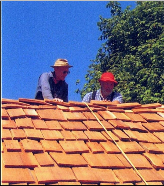
Fig. 36 – Vernon Jenkins, left, and Don Hagen install the last shake on the Barker Cabin roof, July 30, 2002. (Courtesy Lvnda Jenkins. HSFW.)
