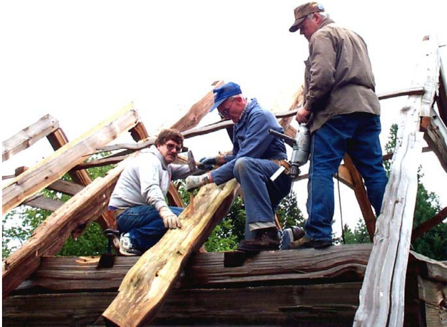
Volunteers working on roof for Barker Cabin restoration
